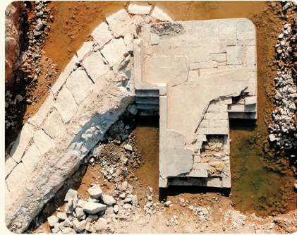
石橋向海末端和海堤 Seaward end of the Bridge and seawall
