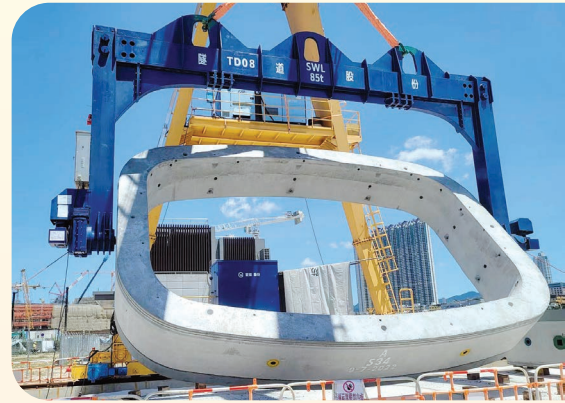
預製組件遙控自動翻身架 Remote automatic turning device for the turning of prefabricated segments
